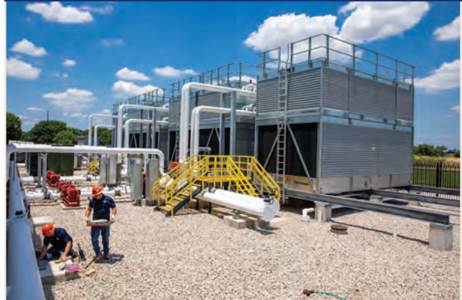
PHOTO 3 Closed circuit cooling towers being installed on a liquid-cooled data center in Houston. Courtesy of DownUnder GeoSolutions
